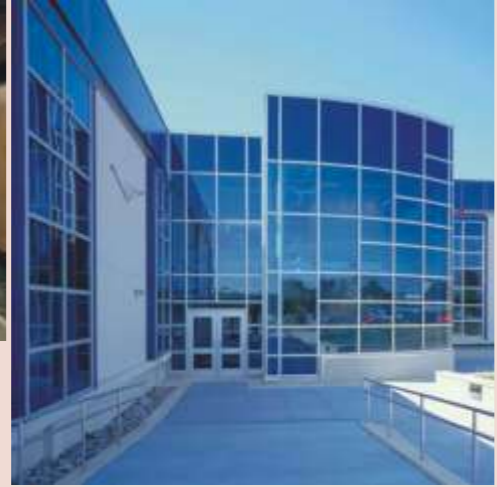
SABARU: US Operations Headquarters. Size: 65,000 SF
