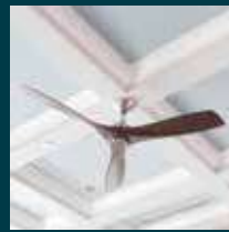
CEILING ACRYLIC EMULSION PAINT/ OIL BOUND DISTEMPER
