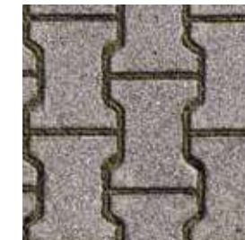
INTERNAL ROADS INTERLOCKING BLOCKS/ TREMIX CONCRETE ROAD
