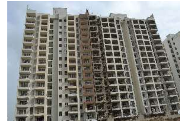
Navodaya - construction photograph
